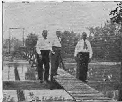
Supt. C. L. Whiting, Divn. Engr.; T. H. Strate and Asst. Genl. Manager, N. A. Ryan Inspecting Bridge Erected by 108th Engineers at Camp Grant.
