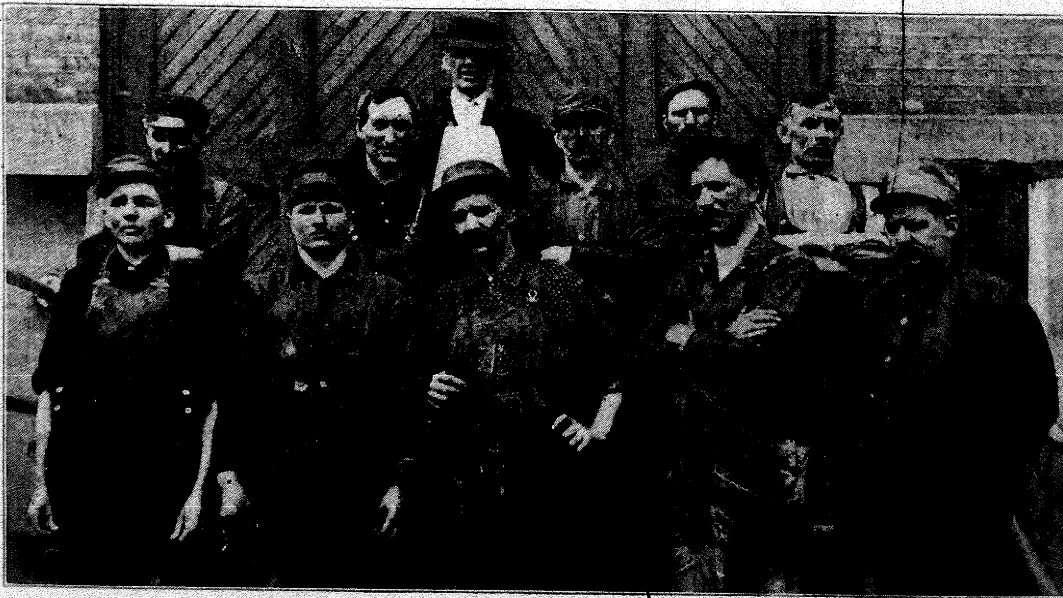
Day Force, Milwaukee Shops Power Plant.
