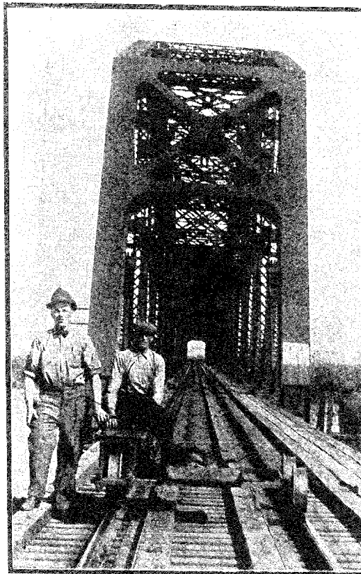
Linemen at the Missouri River Bridge, Mobridge, S. D.
