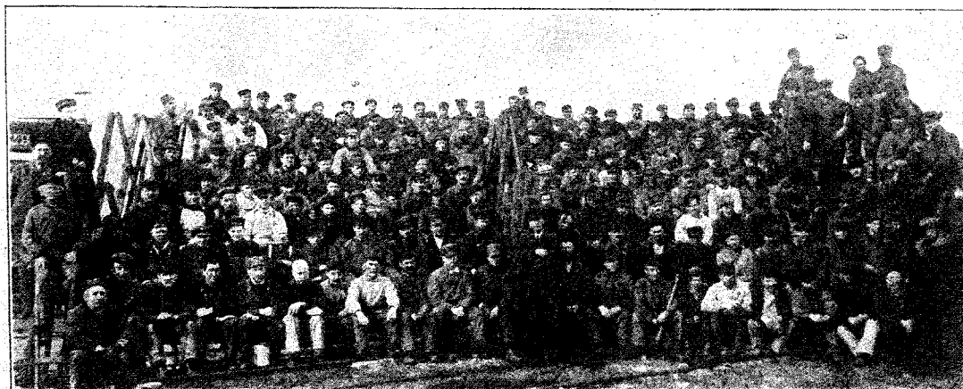
Repair Track Crew, Dubuque Shops.
