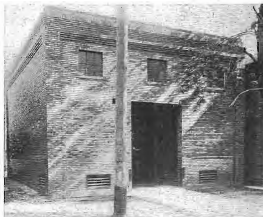
Fig. 6. Automatic Railway Substations (12th and High Streets), Des Moines City Railway Company
