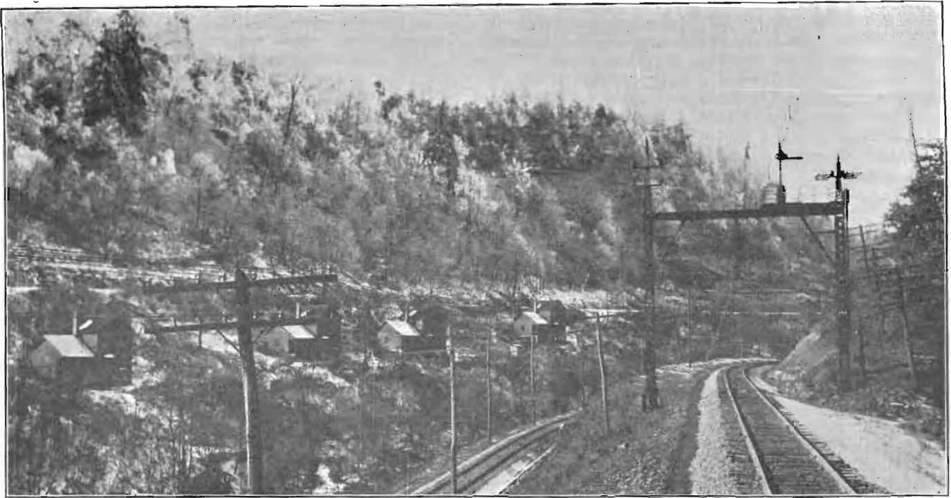
About a Mile East of the Elkhorn Tunnel on the Norfolk & Western
