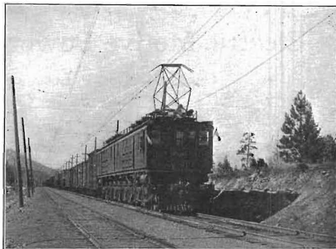
A C. M. & St. P. Freight Locomotive with a 100-Car, 5,000-Ton Train, Eastbound at Thelma on the Missoula Division
