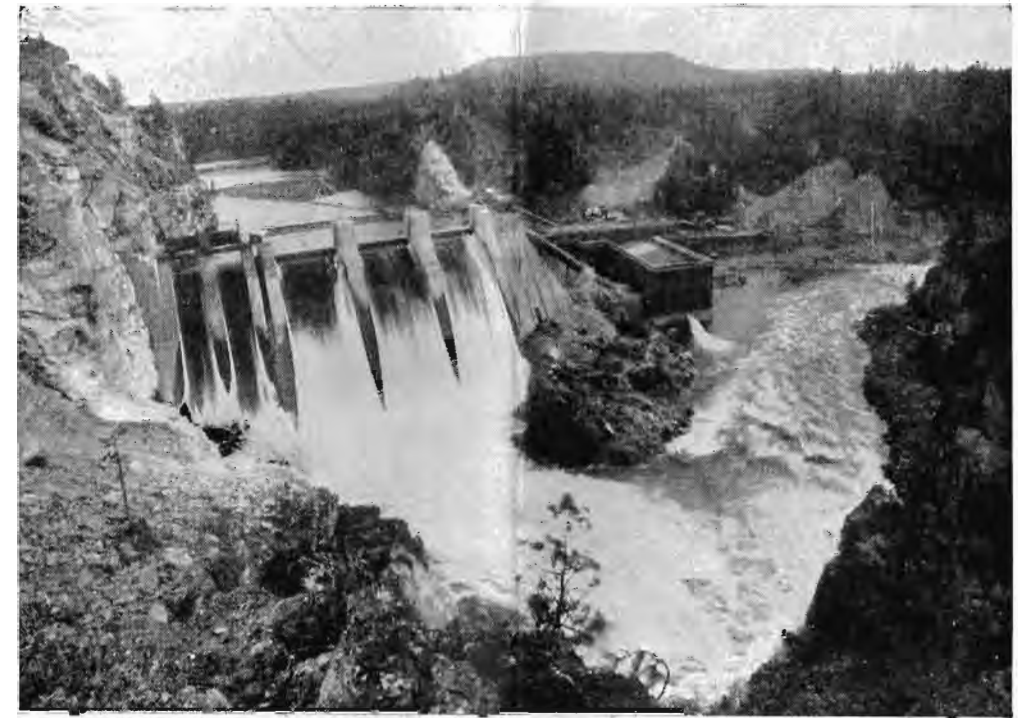
LONG LAKE PLANT OF THE WASHINGTON WATER POWER COMPANY HAVING A TOTAL CAPACITY OF 65,000 HP.
