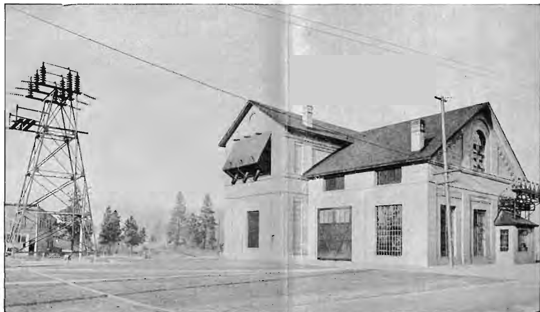
CLE ELUM SUBSTATION
