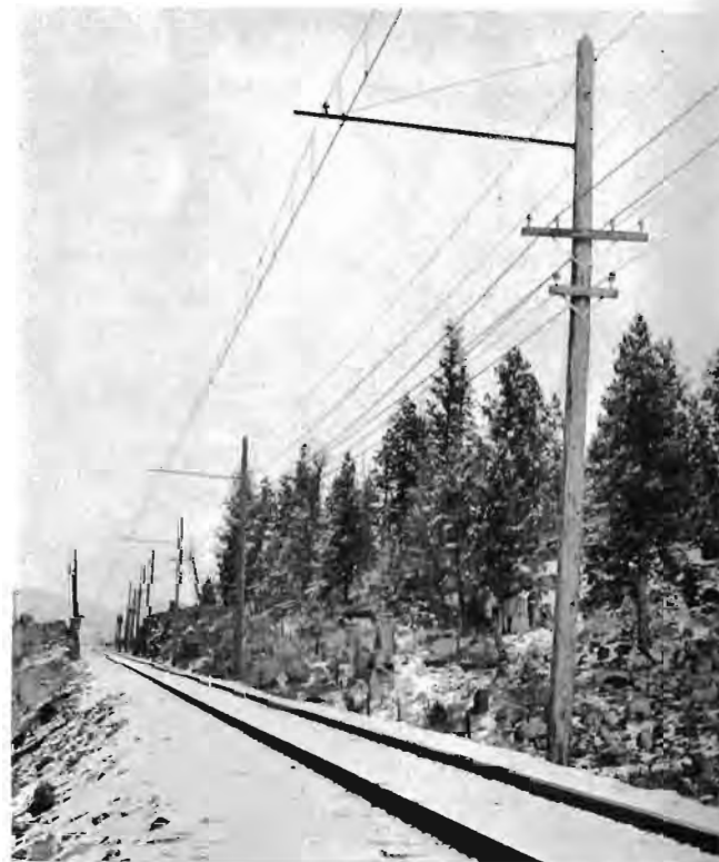
TANGENT BRACKET TROLLEY CONSTRUCTION
