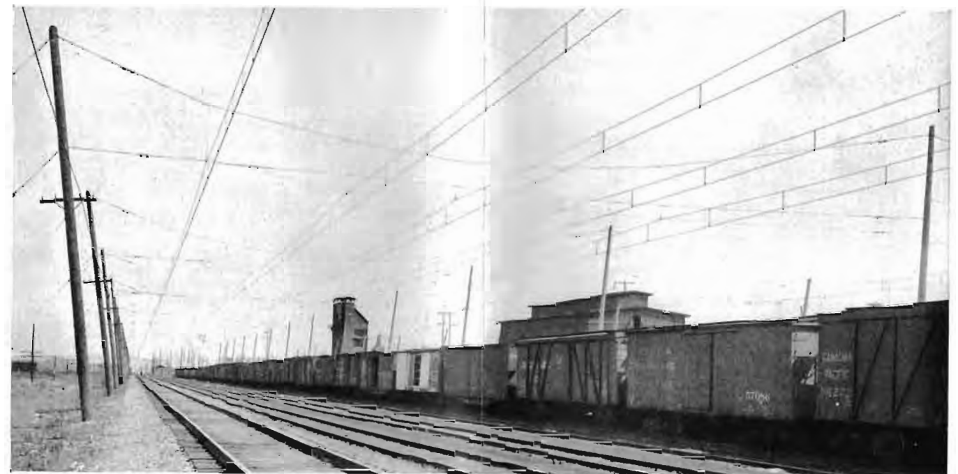
CROSS SPAN OVERHEAD YARD INSTALLATION
