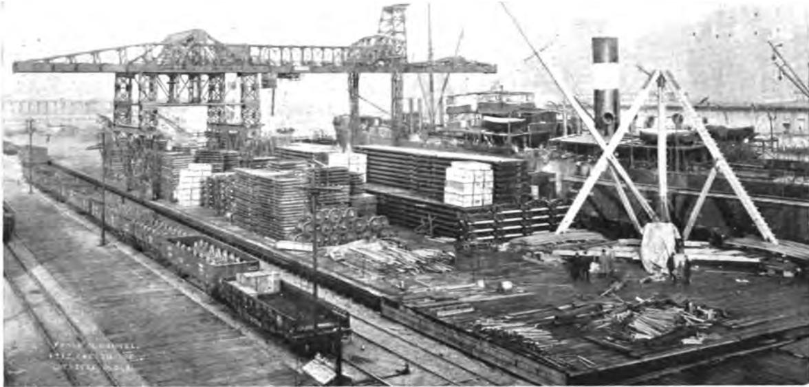
The Smith Cove terminals. Showing handling equipment consisting of a five-ton gantry crane, a fifteen-ton stiff leg derrick and two locomotive cranes.
