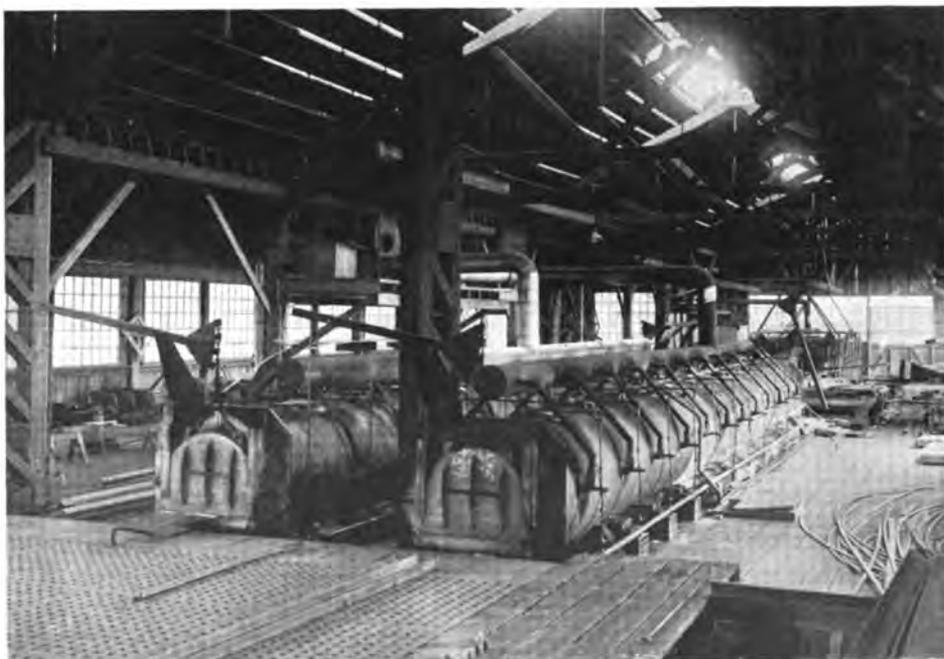
Sectional angle furnaces and a portion of the slab-bending floor at the J. F. Duthie & Company plant.
