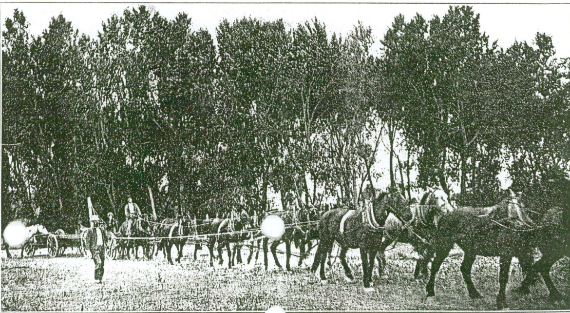
Fig. 32—Typical Freighting Outfit for Forwarding Materials on Construction of Great Falls Line, C. M. & St. P. Ry.
