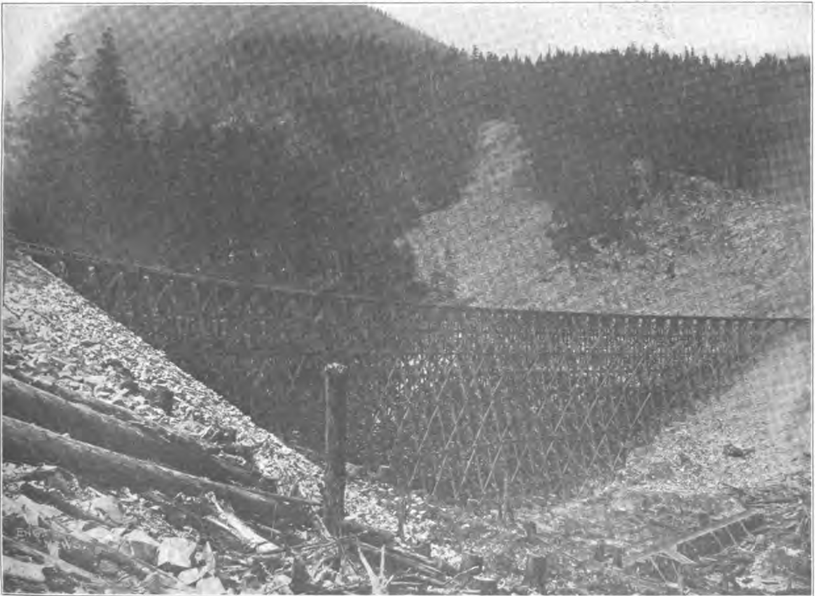
THE MINE CREEK TRESTLE, C., M. & ST. P. RY. (155 FT. HIGH, 1,250,000 FT. B.M. TIMBER).
