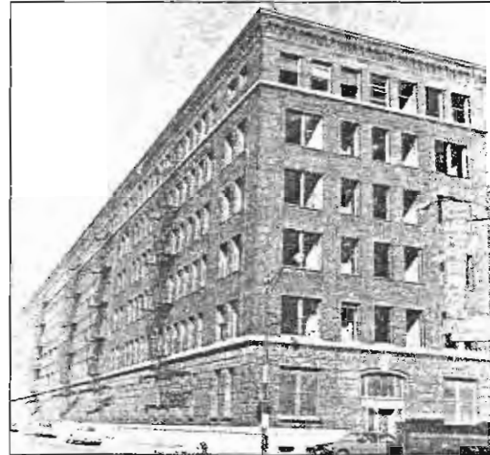
The once-vacant Milwaukee Road building at 2437 N. Southport will become an innovative health care facility. A 20% federal tax credit given to buildings older than 40 years makes renovation a very attractive option.
