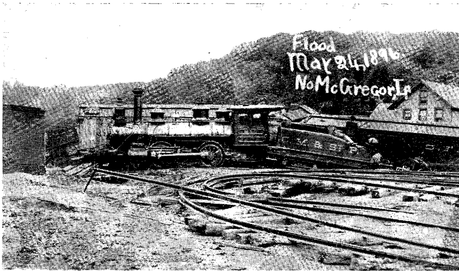
THE RAMPAGE OF 1896. J. E. Bergemeyer, retired B&B foreman now living at Highland, Calif., would like to know how many recall this scene at North McGregor, Ia. (now Marquette), on May 24, 1896, after a flood had washed out the line to Monona. The building in the background at the right is the Rudde Hotel.
