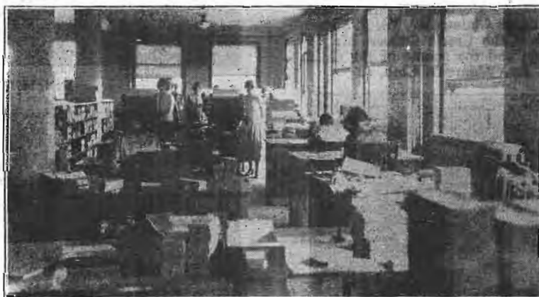
Machine Room, Freight Auditor's Office.
