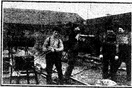
Shows portable oil rivet heater used in repair yard for steel car repairs. Men at work reassembling a C., M. & St. P. 100,000 capacity flat after being wrecked.
