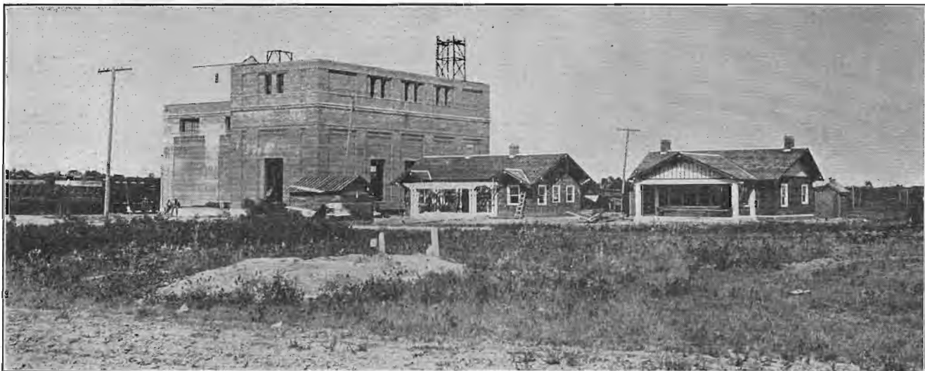
CHICAGO, MILWAUKEE & ST. PAUL ELECTRIFICATION—SUBSTATION AND OPERATORS' HOUSES AT TWO DOT, NEAR THE EASTERN END OF THE ELECTRIFIED DIVISION
