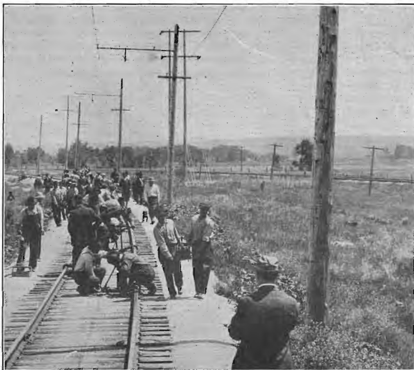
CHICAGO, MILWAUKEE & ST. PAUL ELECTRIFICATION—BONDING CREWS AT WORK—RADIATOR TYPE, 100,000-VOLT TRANSFORMER
