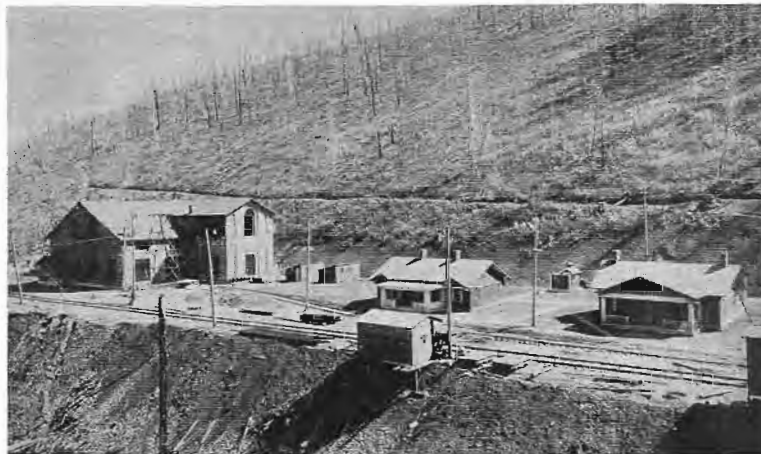
Fig. 4. East Portal Substation with Operators' Bungalows, C., M. & St. P. Station Contains Three 2000-kw. Synchronous Motor-generator Sets
