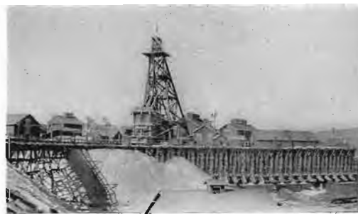
HOIST AND STORAGE BINS ON BUTTE HILL
