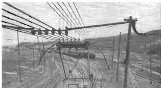
PANTOGRAPH ENGAGING SIX TROLLEY WIRES
