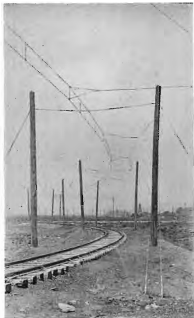
OVERHEAD CONSTRUCTION ON SINGLE TRACK CURVE
