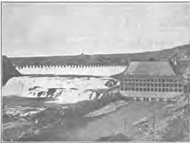
The Great Falls Plant of the Montana Power Co. Capacity 60,000 K.W.
