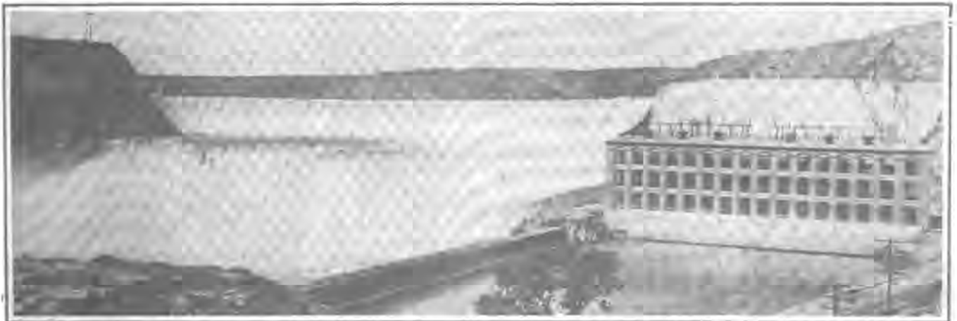
Power House and Dam at Great Falls, on the Missouri River; power being transmitted by the Montana Power Co. to the Chicago, Milwaukee & St. Paul Railway electrification
