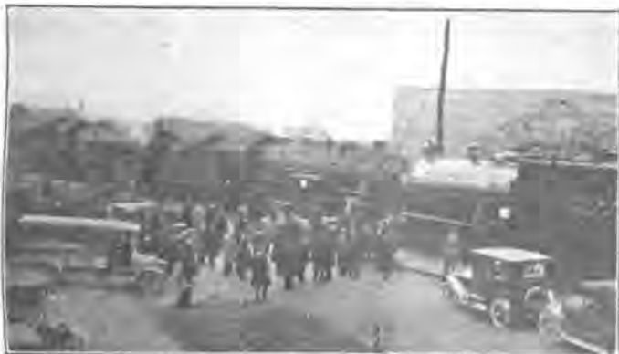
Two Steam Locomotives Used to Supply Power which was Regenerated to the Trolley by the Electric Locomotive
