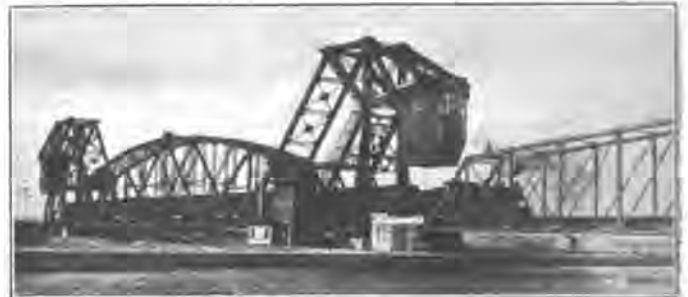
Train Crossing the Bascule Span and Entering the Swing Span.
