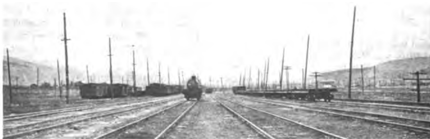
Fig. 23. Section of Tangent Track, showing Pantograph Trolley Suspension as sketched in Fig. 17
