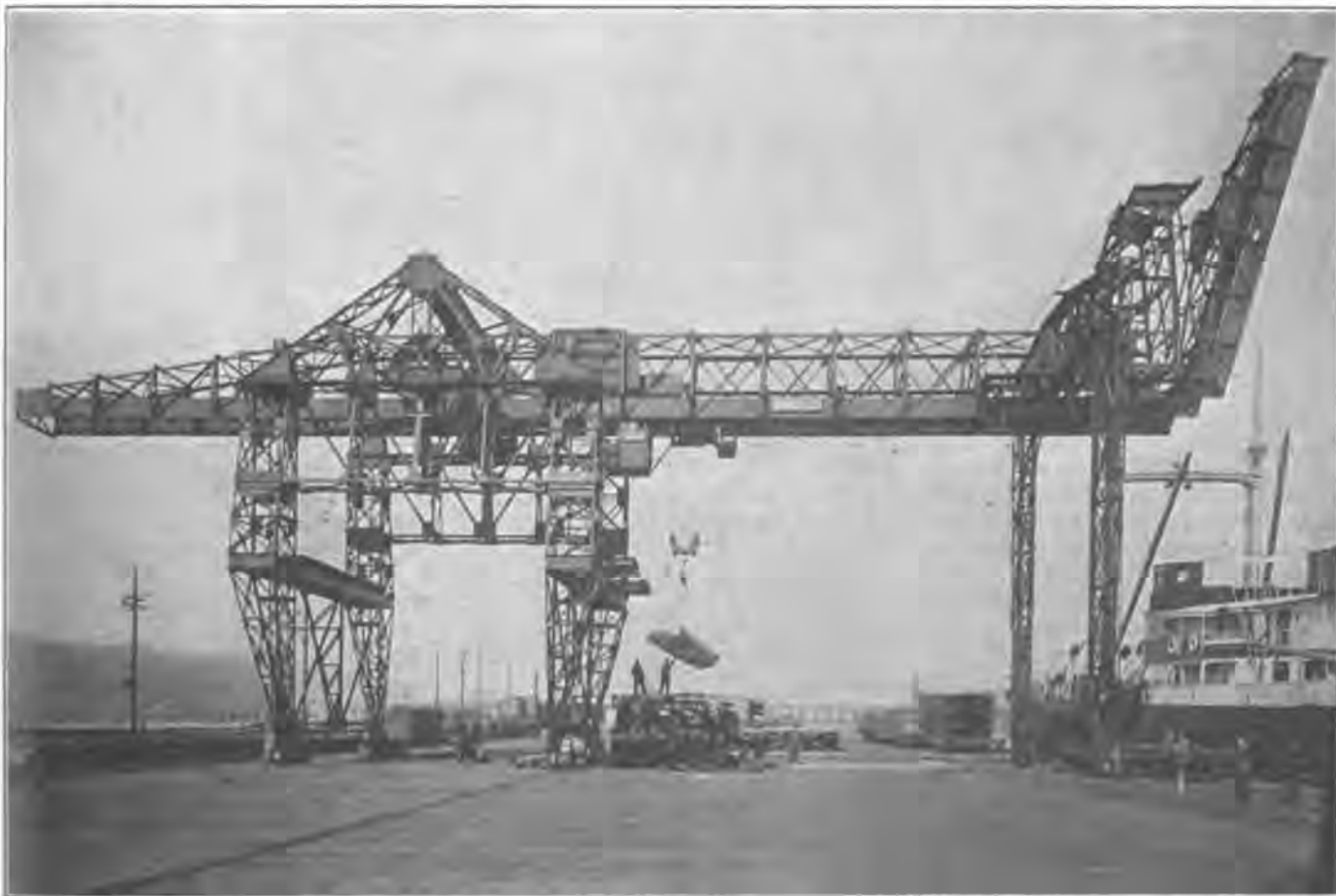
Great traveling crane used on the Seattle piers—lifts 65 tons, carries 30 tons Courtesy of Manning, Maxwell and Moore
