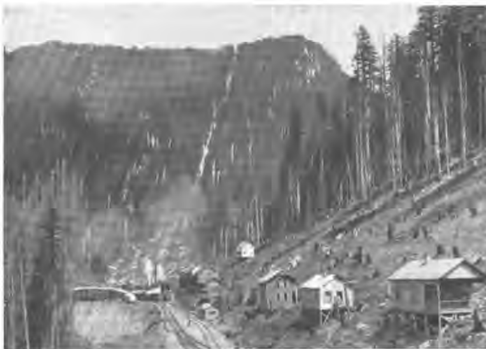
THE ROCKDALE SIDE OF SNOQUALMIE TUNNEL
