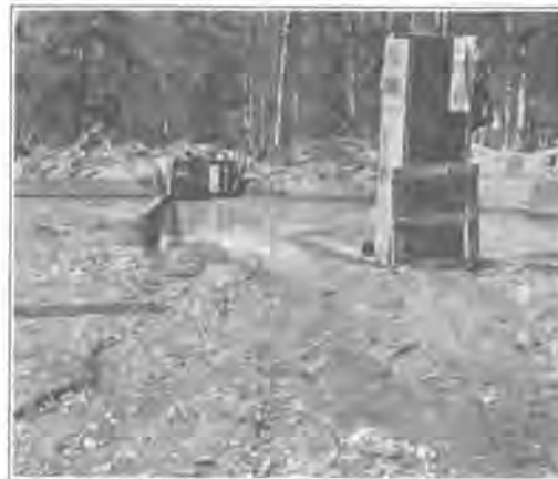
Fig. 10. Vertical Drain or "Chimney" for Draining Water from the Settling Pool Through the Bank.
