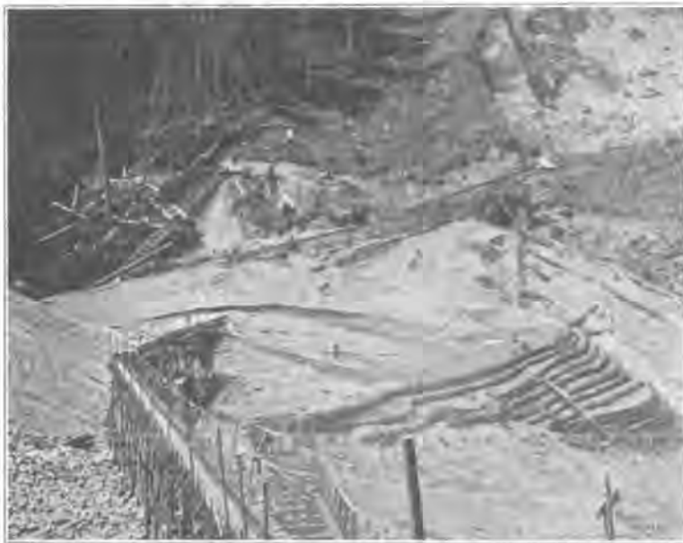
FIG. 8. HYDRAULIC EMBANKMENT AT TOPOGRAPHER'S GULCH; C., M. & ST. P. RY.
