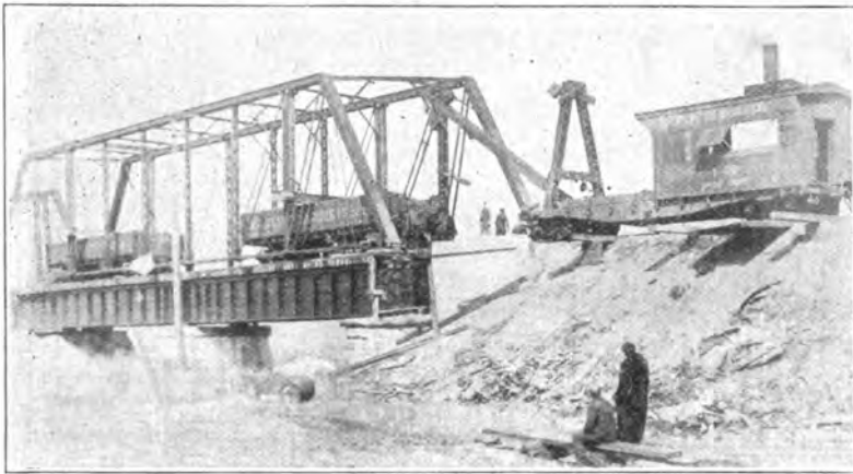
Replacing Trusses with Girders, Pere Marquette R. R.
