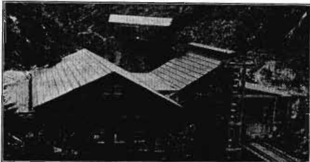
General View of the Ventilating Plant with the Power House in the Foreground and the Fan House in the Rear
