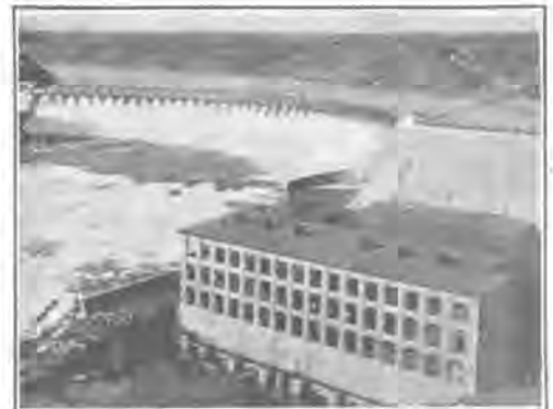
Where Water Power is Turned Into Electricity for the St. Paul Road
